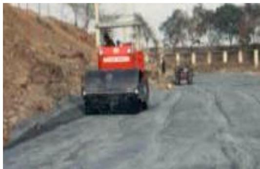
**Figure 3.3.4-13: Vibrating roller working on compacting**
