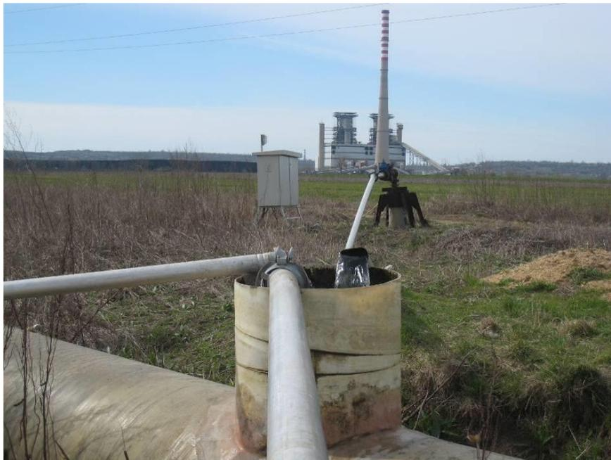
**Figure 2.8-2: Decreasing level of groundwater by a network of drainage wells**
