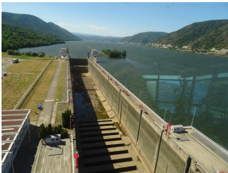
Figure 3.4 - Navigational lock "Djerdap I", upstream fore-dock, lower head and upstream chamber
