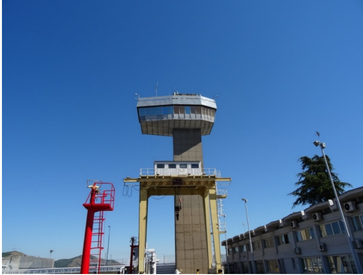
Figure 3.6 - Navigational lock "Djerdap I", command tower
