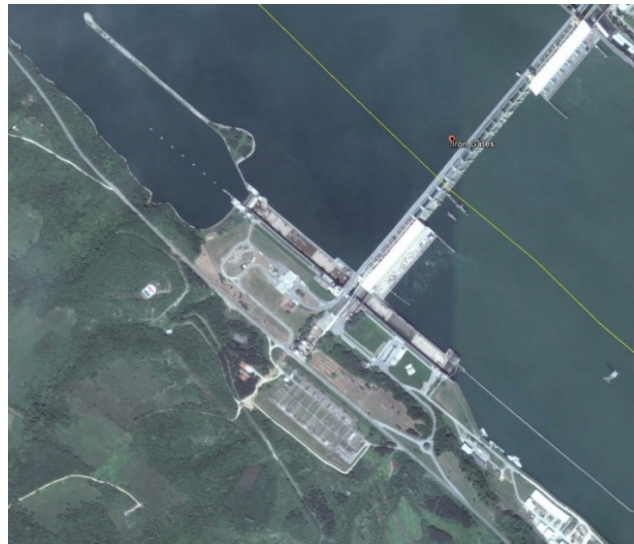
Figure 3.3 - Navigational lock "Djerdap I", right bank
