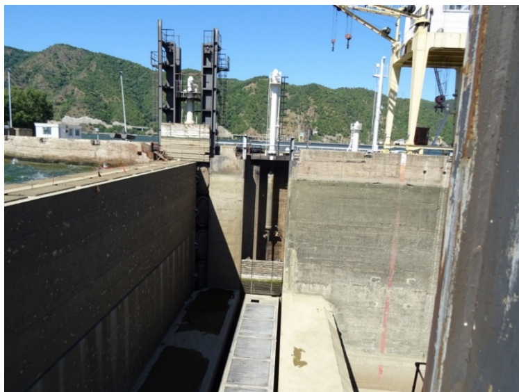
Figure 3.8 - Navigational lock "Djerdap I", upper head, overhaul-repair (in operational position) and main operational door (in the niche)
