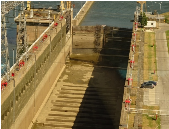
Figure 3.10 - Navigational lock "Djerdap I", lower head, overhaul double door
