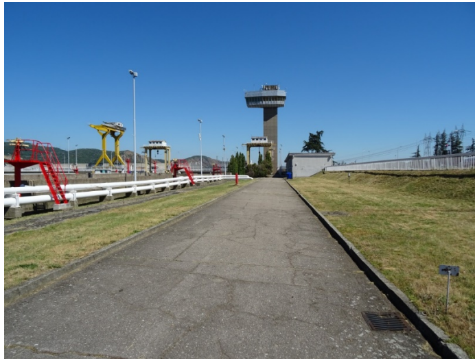
Figure 3.12 - Navigational lock "Djerdap I", portal cranes
